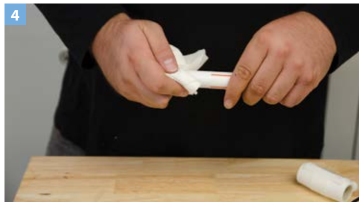
4) Clean pipe ends with an approved aquatechnik ® cleaning solution or isopropyl alcohol wipes.
