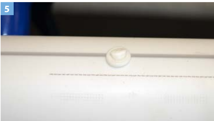
5) Cut the excess material off of the plug.
