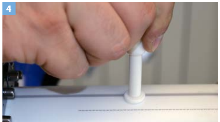
4) Insert the plug stem into the hole and wait for the weld to cool.
