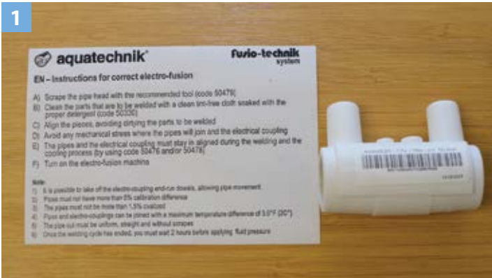
1) Remove electro-fusion fitting from the package and read the instructions in their entirety. Note: Fittings should be left in their packages until ready to use as electro-fusion fittings are more sensitive to contaminants and may not fuse properly if they are not clean.
